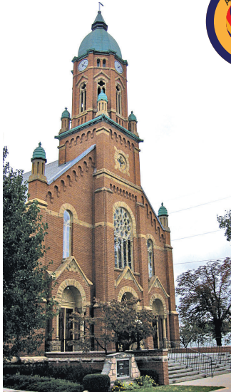
Built in 1895, many features of Defiance St. John the Evangelist are original to the church, including the stained glass windows, high altar, steeple bells, Stations of the Cross and statues. Chronicle photo by Andrea Slivka
